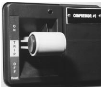
Circuit Breaker Handle Mechanism
