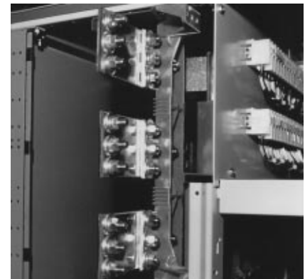
Horizontal Bus Splice Bars
