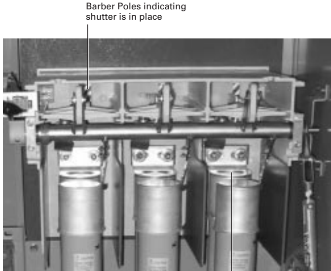
Blown Fuse Indicating Device
