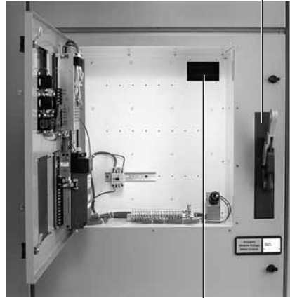
Isolated Low Voltage Control Panel
